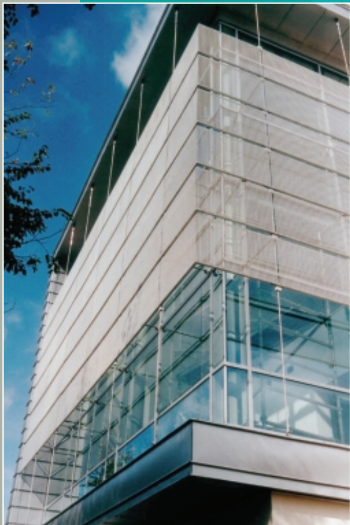
Above: Centre For Power Transmission & Mission Control, Bath University, Bath
